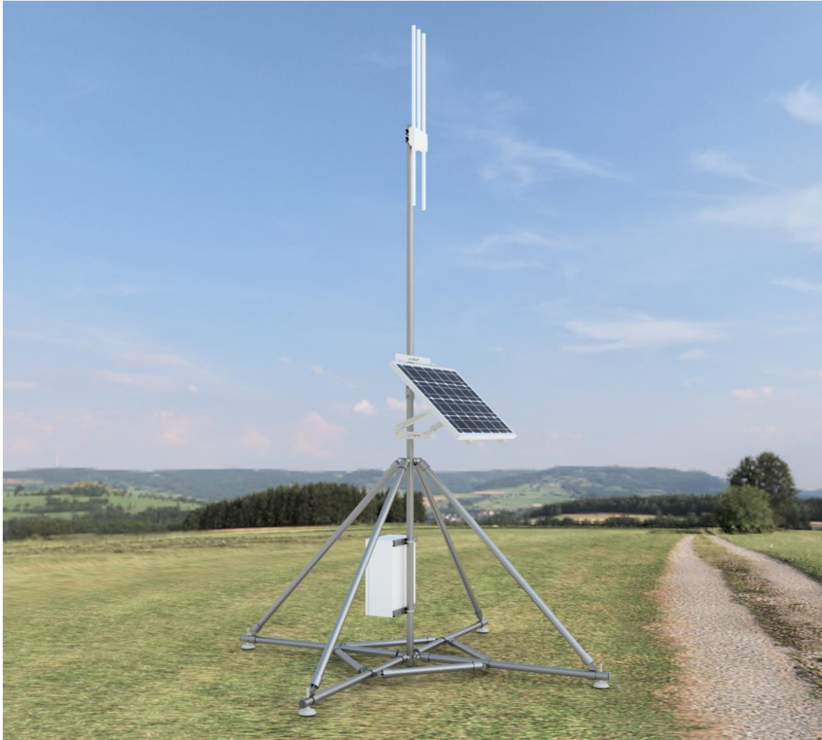
Figure 1: Solar Powered Gateway installed on-site
